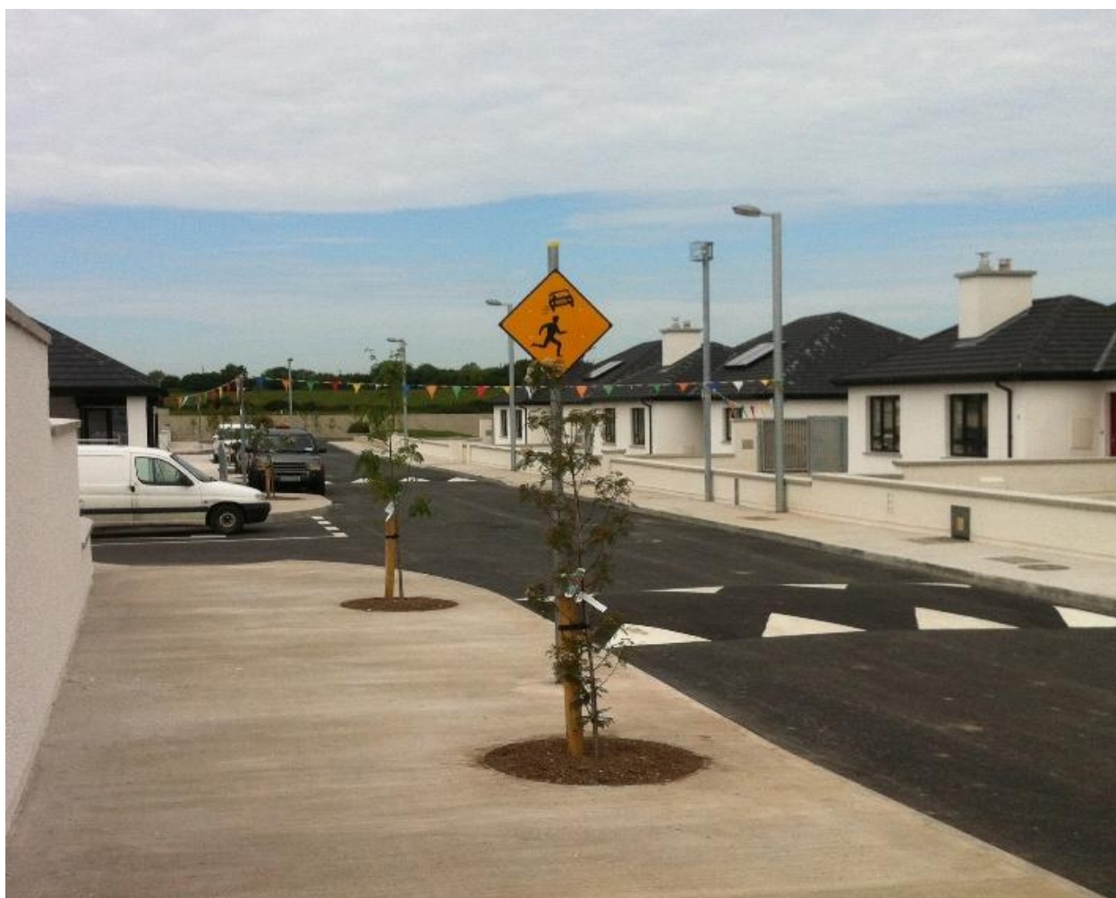
The new group Housing Scheme in Holyhill.
