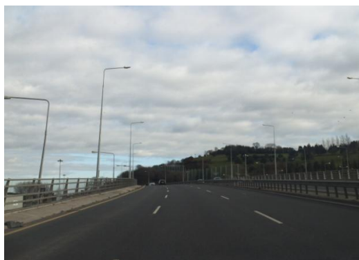
Street view of the grade separated overpass.
