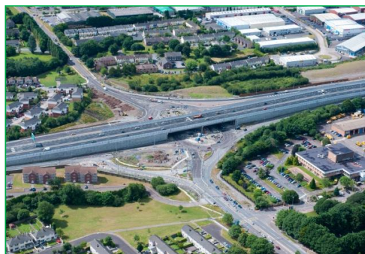
Aerial view of project under construction
