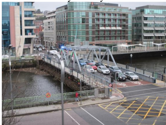
Clontarf Bridge, December 2015, prior to demobilising suspended scaffolding to bridge footways.
